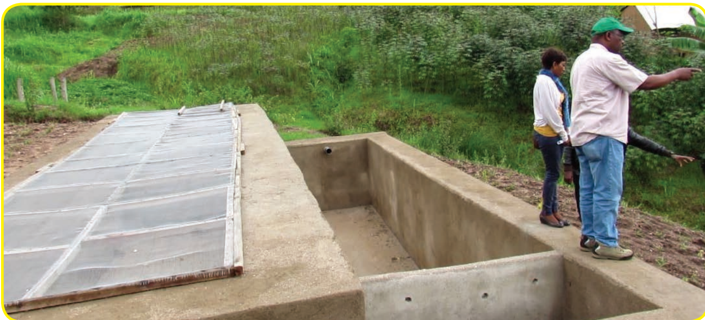
ARCOS team visits Sholi to assess the activities of the construction of the water treatment Phot: ARCOS
